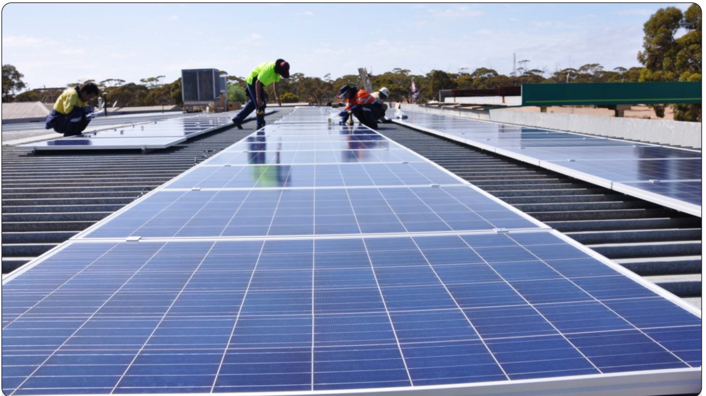
Rooftop solar panel installation
